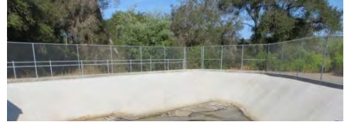
Figure P-9.1.003 Raceway Basin Pump Station Existing Fence
