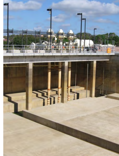
Figure P-9.5.005 Carlsbad Water Recycling Facility EQ Basin
