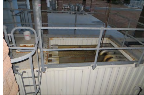
Figure P-9.5.002 Carlsbad Water Recycling Facility MF Modules
