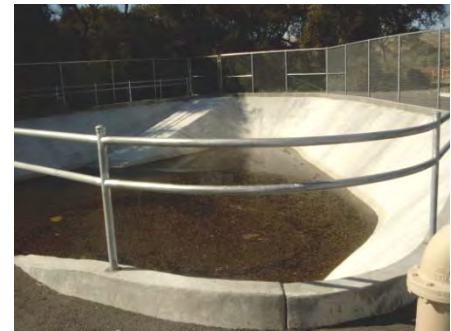
Figure S-9.1.001 Raceway Basin Pump Station Containment Basin
