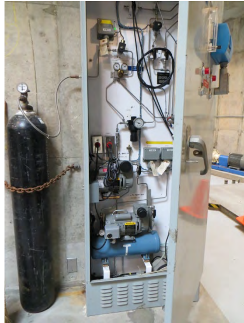
Figure P-9.3.002 Buena Vista Pump Station Bubbler System
