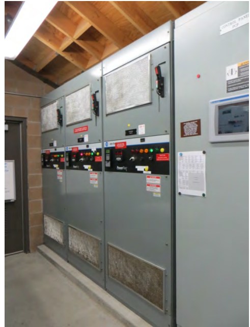
Figure P-9.1.004 Raceway Basin Pump Station PLC Units
