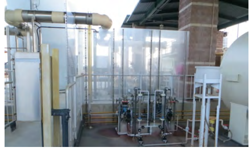
Figure S-9.5.004a Carlsbad Water Recycling Facility Sulfuric Acid Feed System
