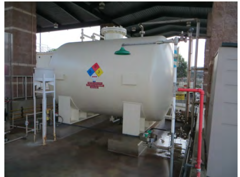
Figure S-9.5.004b Carlsbad Water Recycling Facility Sulfuric Acid Storage Tank
