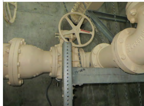
Figure P-9.4.001b Buena Creek Pump Station 8-inch Discharge Plug Valve
