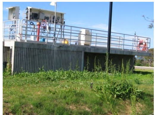
Figure P-9.5.001a and b Carlsbad Water Recycling Facility Chlorine Contact Basin
