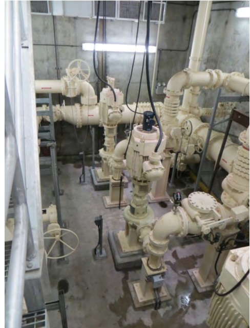
Figure P-9.4.001a Buena Creek Pump Station Pump Room Overview
