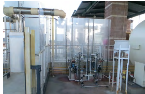
Figure P-9.5.004a Carlsbad Water Recycling Facility Sulfuric Acid Feed System
