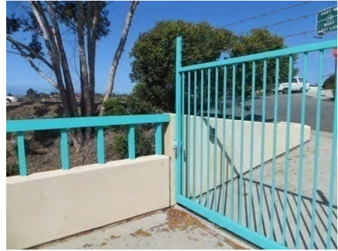
Figure P-9.3.007 Buena Vista Pump Station Security Fence Modifications
