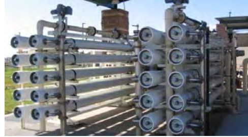
Figure P-9.5.003 Carlsbad Water Recycling Facility Reverse Osmosis Modules
