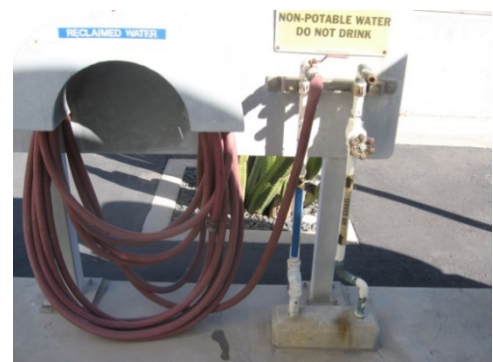
Figure 5-20: P-5.2.017, Service Air/Washdown Station
