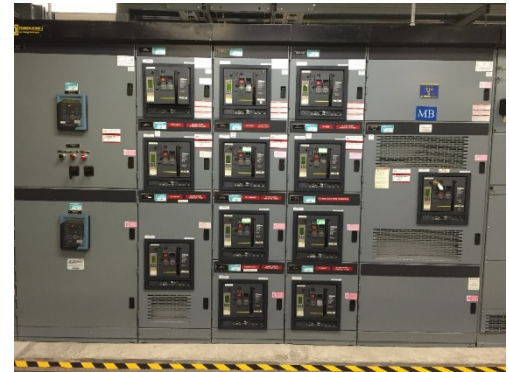
Figure 5-16: P-4.1.024, Main Breakers at Cogen
