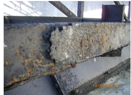
Figure 5-4: P-1.3.007, Secondary Clarifier Nos. 5, 6, & 8 Corrosion
