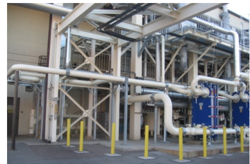
Figure 5-14: P-4.1.012, Plated Heat Exchangers (in Blue)
