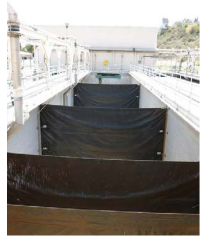
Figure 5-7: P-1.3.018, Example of Geomembrane Baffle
