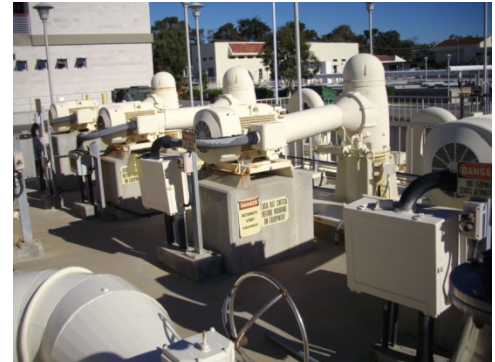
Figure 4-1: P-1.4.001, Final Effluent Pumps
