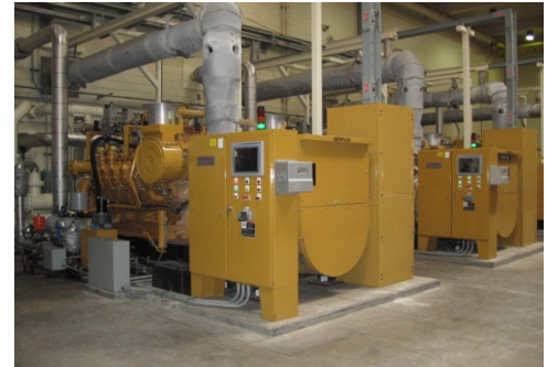
Figure 5-15: P-4.1.015, Cogeneration Engine Nos. 1 & 2
