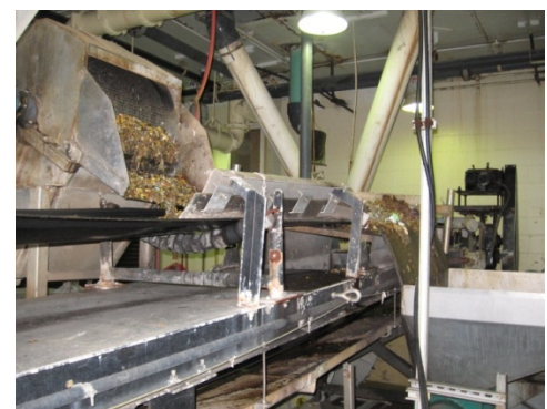
Figure 5-1: P-1.1.005, Bar Screen Conveyor
