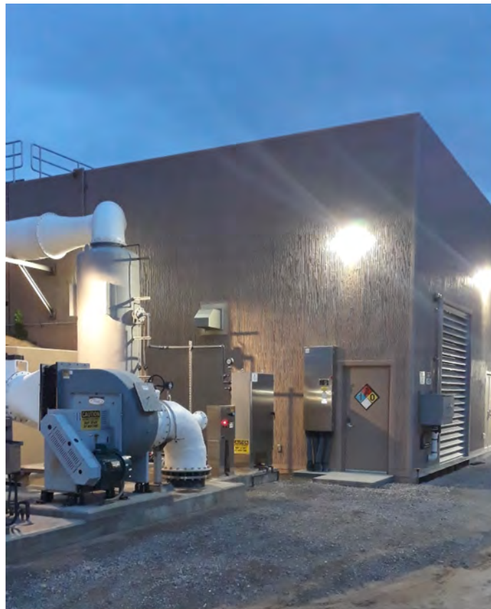
Newly Constructed Agua Hedionda Pump Station
