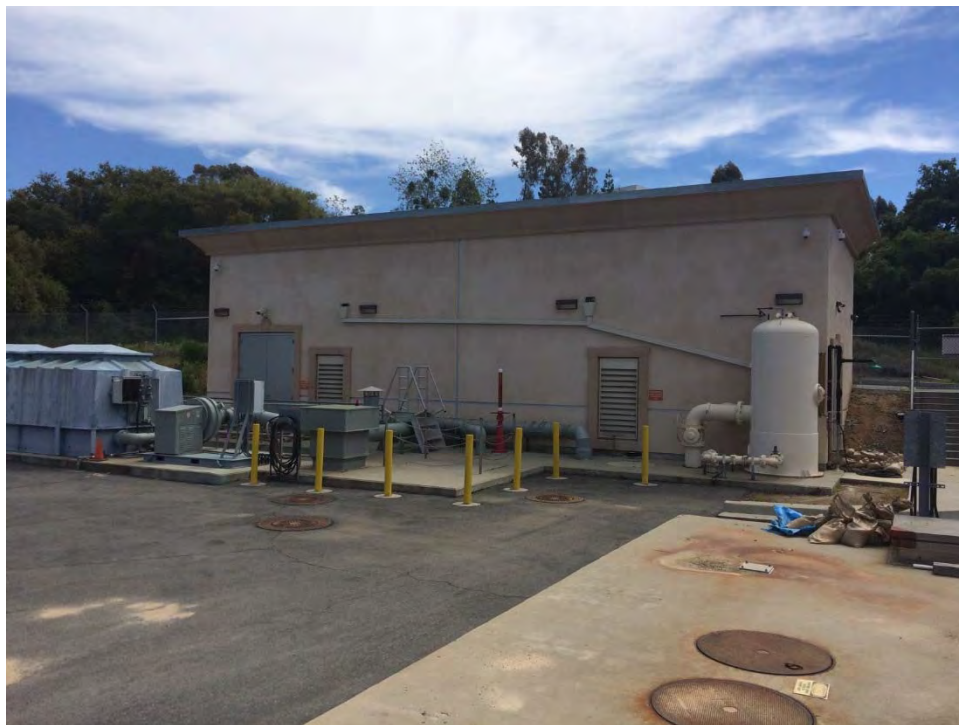
Buena Creek Pump Station
