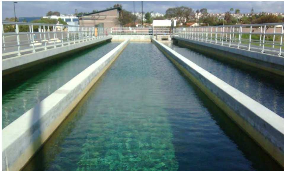
Carlsbad Water Recycling Facility
