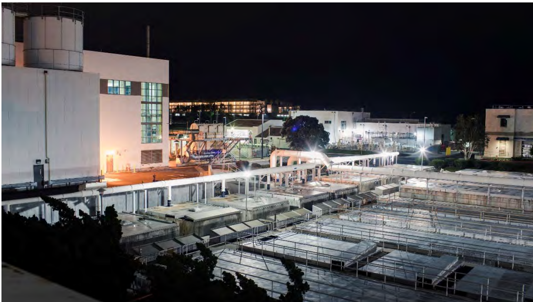
Primary Treatment Area
